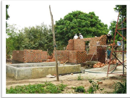
CONSTRUCTION AT JACKFRUIT
